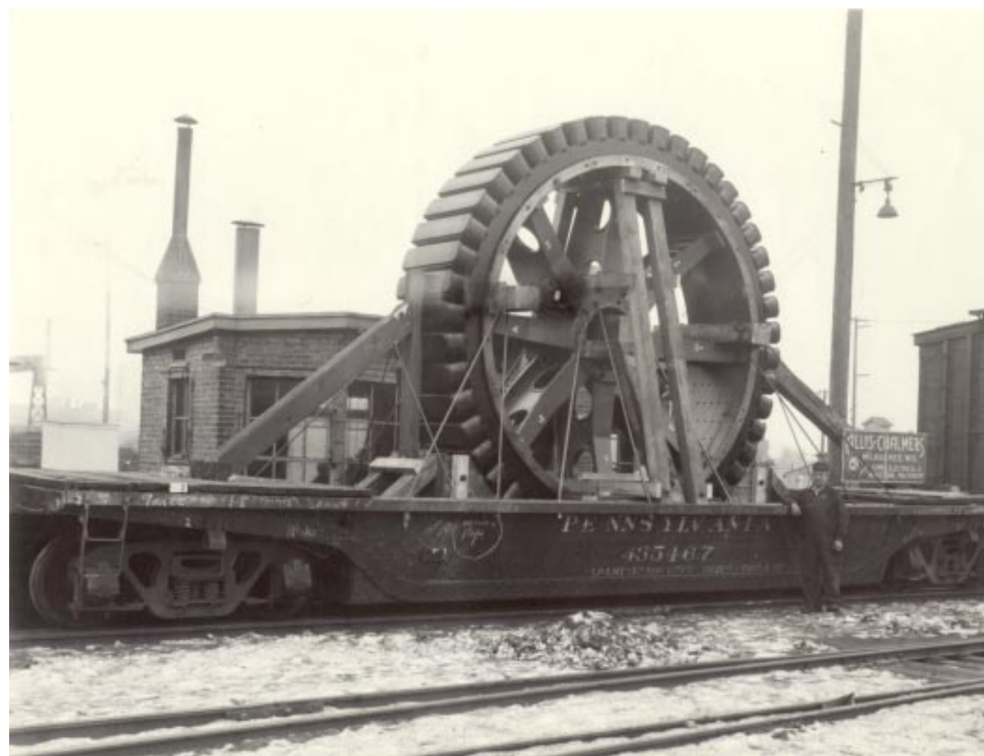
At left, one of the rotors for the project's powerhouses arriving at the Columbus Railroad Depot. Special rail lines were built to the Columbus Powerhouse to haul large equipment like the rotor pictured.
